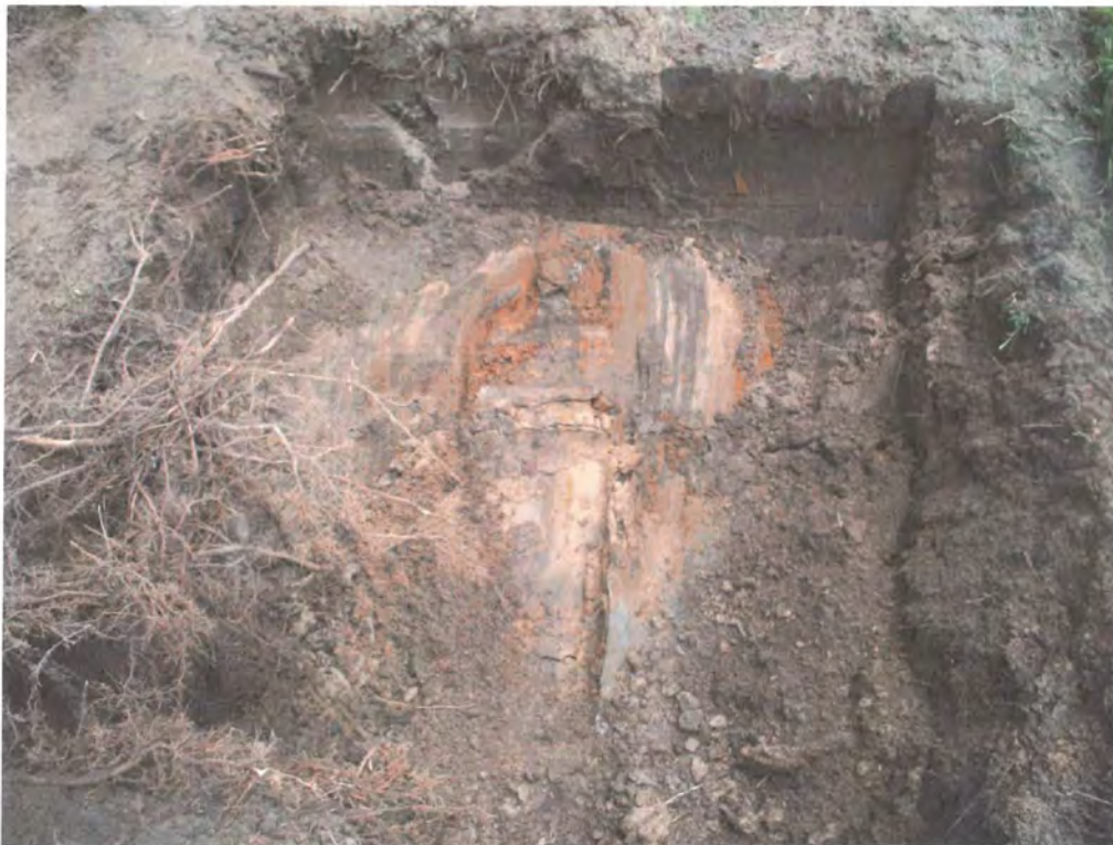
Picture 2: Tank excavation in progress.
